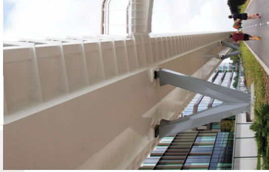
Bridge Pier Options There are a number of options for the abutment pier, depending on architectural intent and budget. Options range from RC columns to V-Shaped piers.
